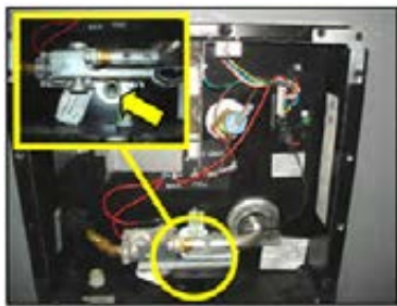
Water heater drain plug location
