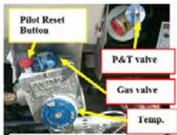
Water Heater pilot ignition
